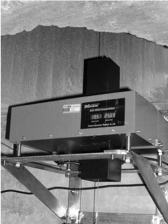
Figure 22 - Light Shields Installed
